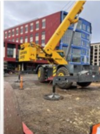
Hoffman Construction hard at work
